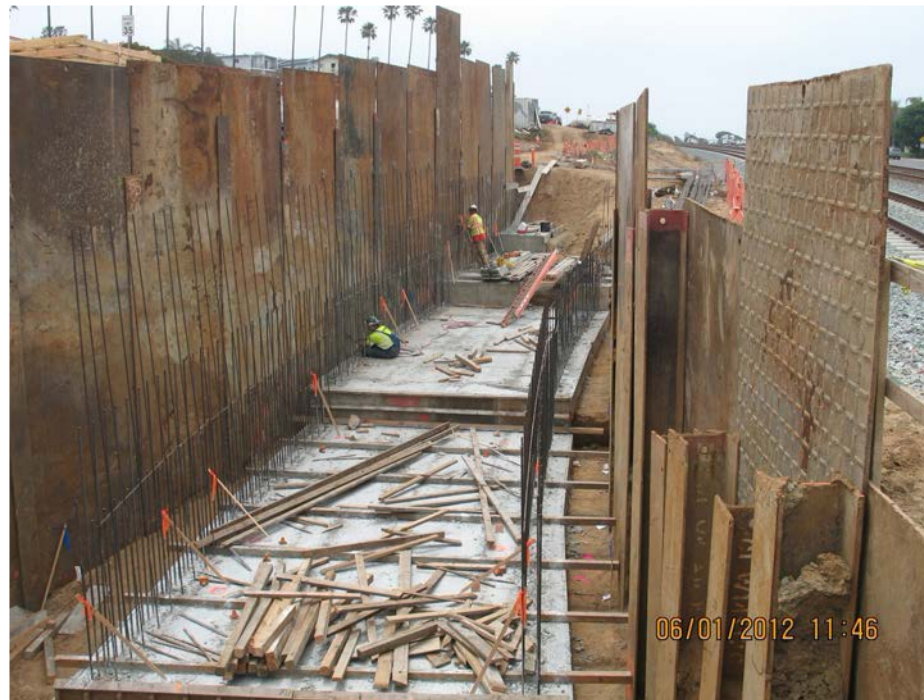
Retaining wall construction
