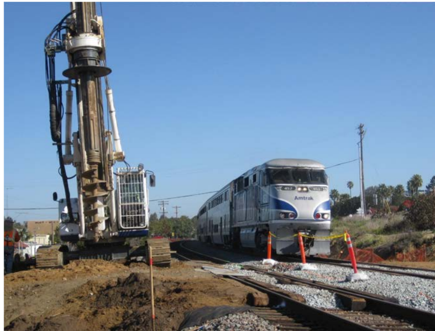
Drilling bridge foundations
